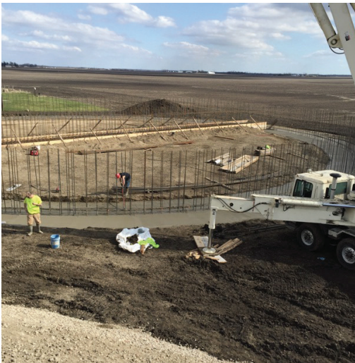
Pump truck pouring the footing of the bin
