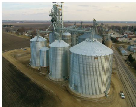
Aerial view of new bins and leg tower
