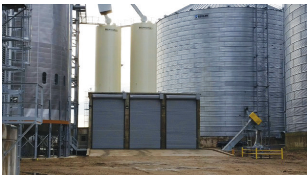
New pit house and gravity tanks
