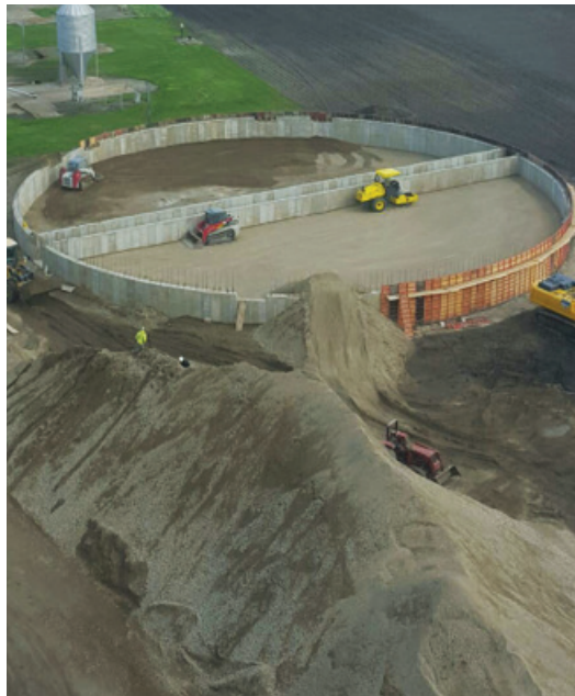
Filling the base of the bin with fill rock.
