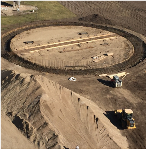
Setting rebar and preparing to pour bin footing
