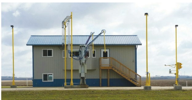
New Office showing the Inbound and Outbound scales and a probe designed and built by GRAINLAND Staff
