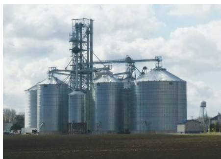
New bins and office
